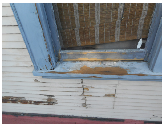
IMB “BEFORE” photos: replacing dry-rotted wood and sealing the exterior was first priority.
